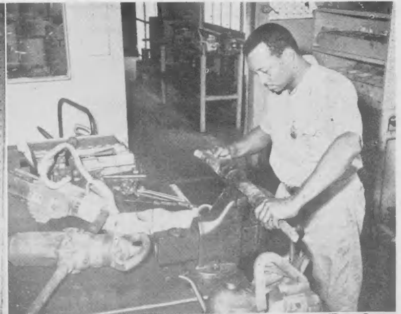
PIPE WRENCHES come in all sizes. The largest is this 48-inch tool. Checking out tools, foreground, is J. Maybelly, one of nineteen tool room employees. YABI DI tubo ta bin den tur tamanjo. Esun di mas grandi ta di 48 duim. Entregando herment, adilanti, ta J. Maybelly, un di e diez-nuebe empleadonan di Tool Room.
